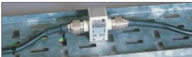
ESP RF 111121 installed on a coaxial cable running between an antenna and an RF receiver. Note the earth lead (behind the cable tray) attached to the mounting fixture.
