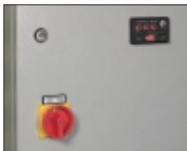
Front view of a cabinet with the display unit, easily visible, mounted on the front of the door, whilst the protector unit is installed deep within.
