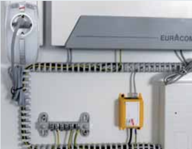
Surge arrester for telecommunications terminal devices and telephone systems with RJ plug-in connection for surface mounting.
