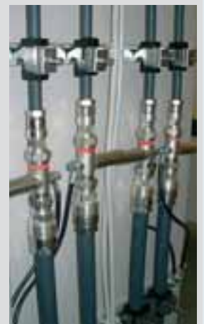
Application of Lambda/4 arresters
